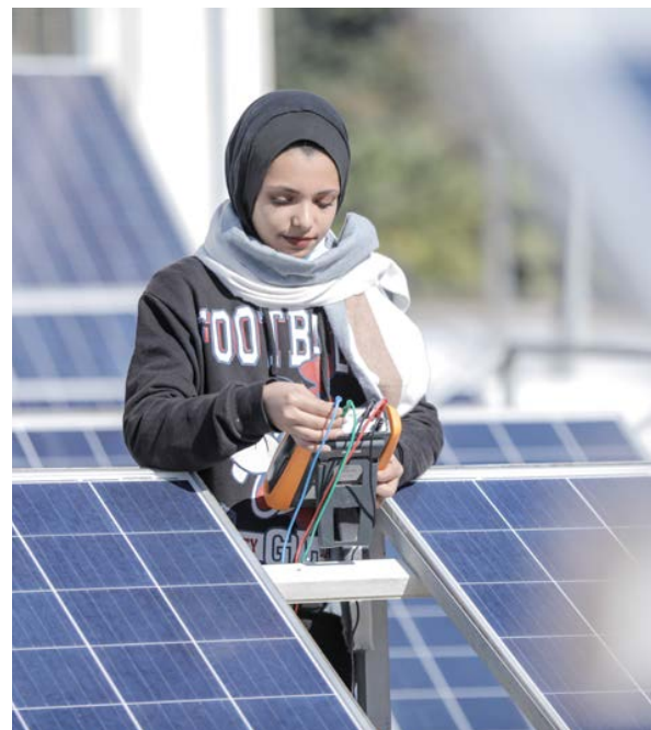
UNRWA's Gaza Training Centre provided vocational training to female and male Palestinian refugees on installing, operating, maintaining and programming solar photovoltaic systems. (2021 UNRWA/ M. Hinnawi)
